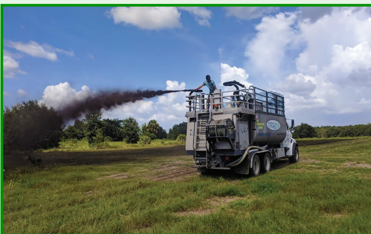
Application through hydroseeder
