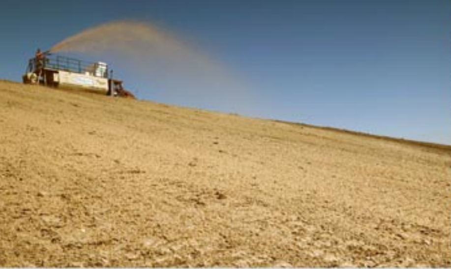
GeoPerm™ applied on 2:1 Slopes
